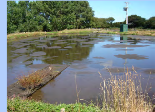
FIGURE 3: Accumulated Biosolids in the Wastewater Treatment Lagoon
