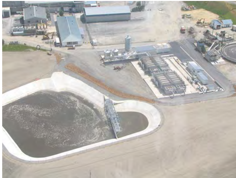
Photograph 2: Overall layout of the Finegand Upgraded Wastewater Treatment Plant
