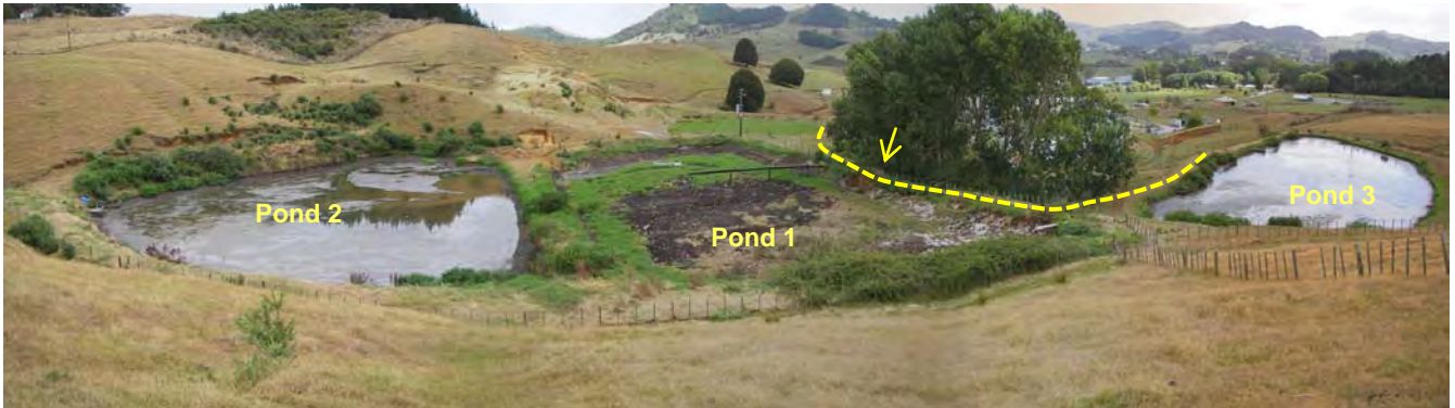
Photograph 2: Anaerobic Lagoon (Pond 1) showing the cracking line and scarp (arrow)
