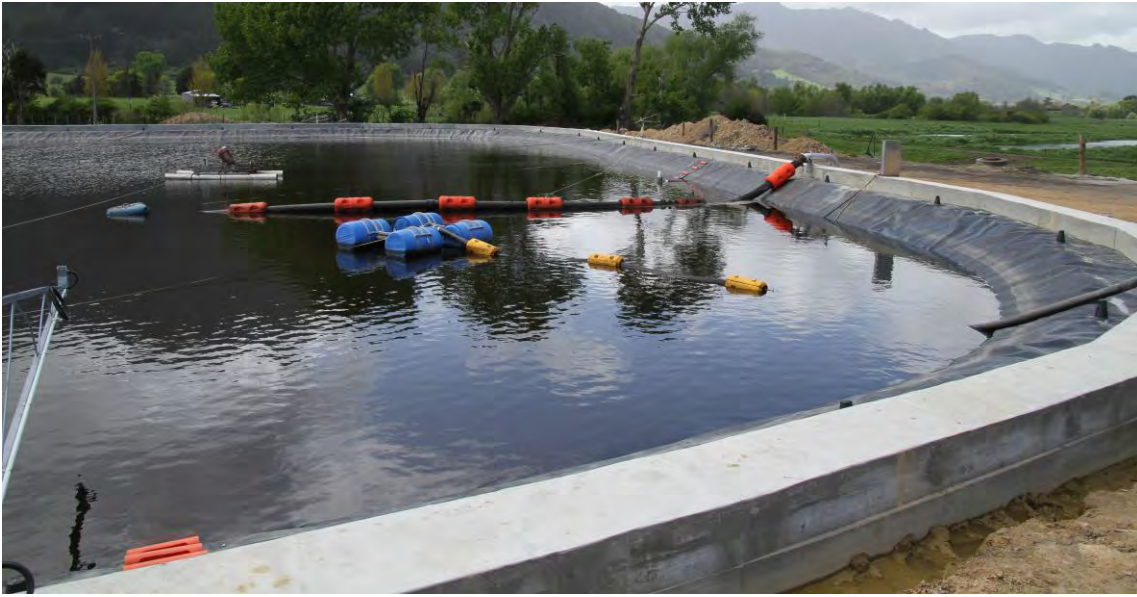
Photograph 6: Completed Relined SBR in Normal Operation
