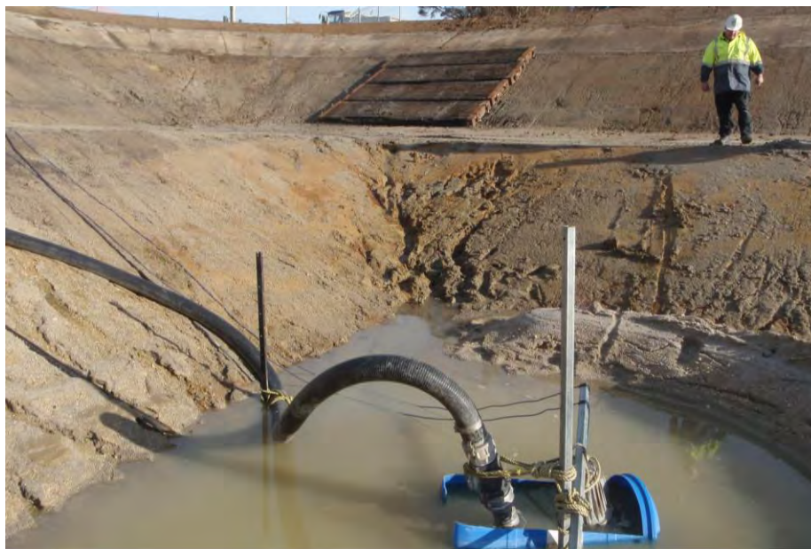
Photograph 3: Dewatering pump working in the low corner of the lagoon base
