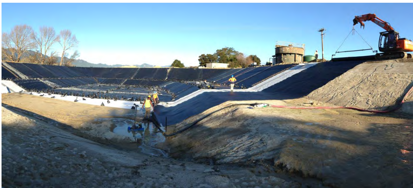
Photograph 5: Relining of the SBR underway
