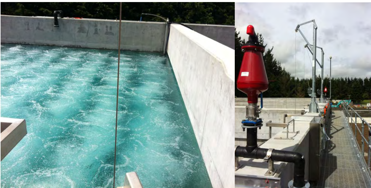
Photograph 2: Water testing of the SBR tanks
