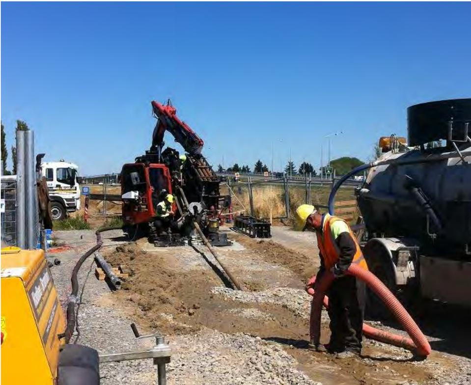
Photograph 1: Directional Drilling Operations
