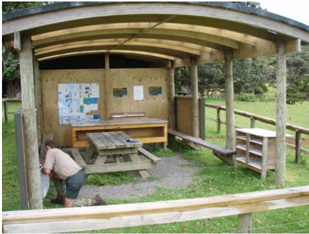
Figure 3. Typical new shelter.
