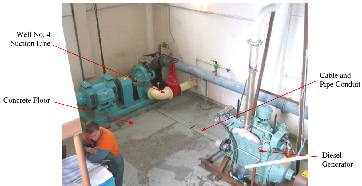
Photograph 3: Inside Pumping Station
