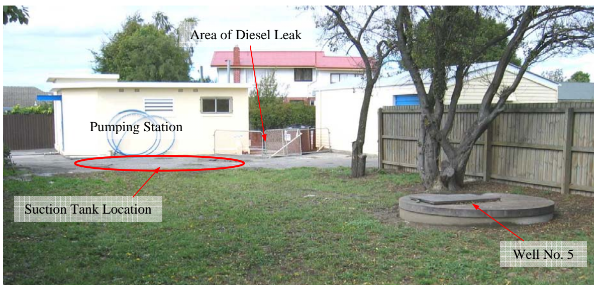
Photograph 1: Auburn Ave Pumping Station (viewed looking east)
