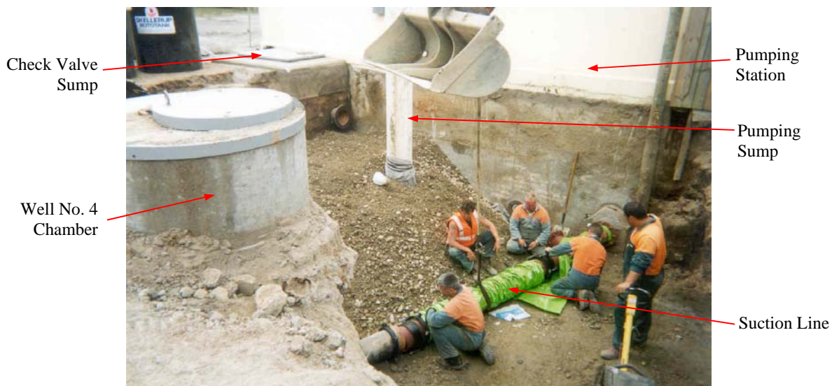
Photograph 2: Excavation to Rear of Pumping Station
